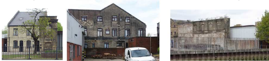
Figure3: showing existing Magnolia House.
