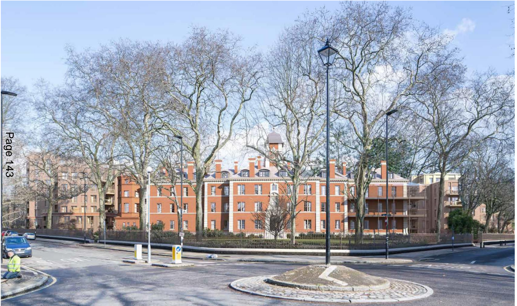
Verified (winter) view from junction of Bonner Road and Approach Road (showing proposed Northern and Southern Buildings set to left and east (respectively) of Main Hospital Building)
