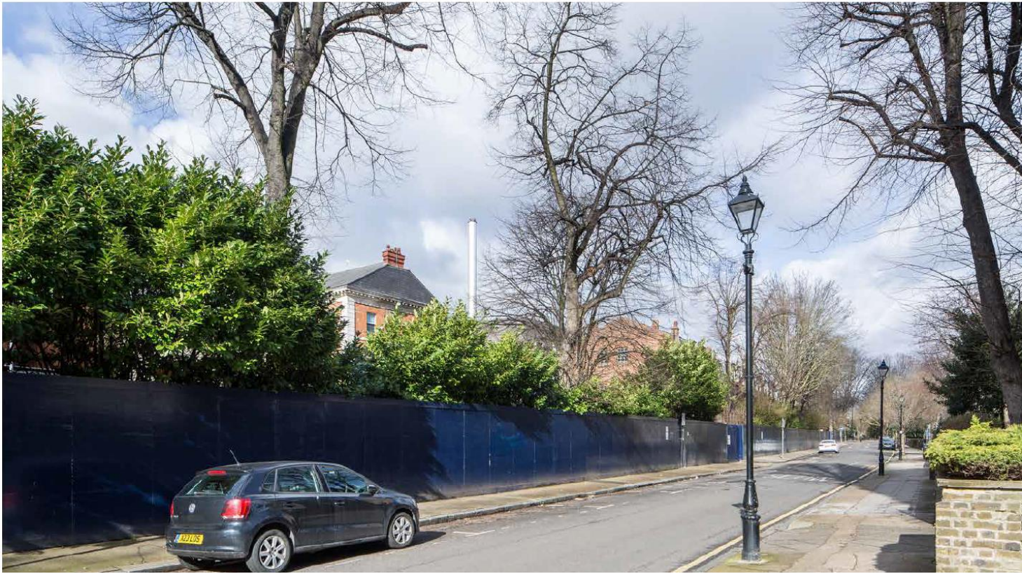
Verified view existing (above) and proposed (below) from St James's Avenue – looking north with proposed South Building (to left) and proposed Central Building (in centre) of CGI
