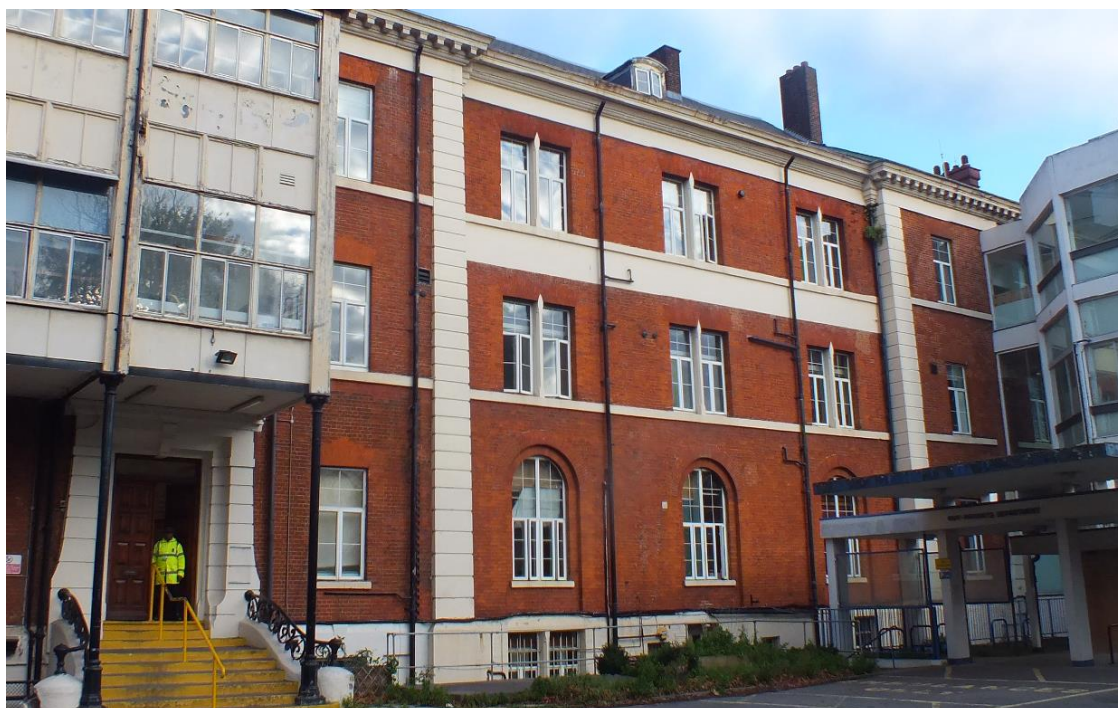
Figure 22: South wing of the hospital building with infilled verandas and new extension
